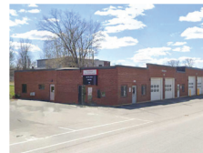
Guilford Guilford Fire Station (GFS) 4 School Street, Guilford
